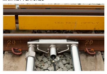
Our PTW allows for greater flexibility without the need to remove rail fastenings due to its length of only 500mm. This results in a more convenient installation and less 'flexing' of the system. The benefits of this are more accurate and reliable weighing results than your ordinary train weighing systems.
