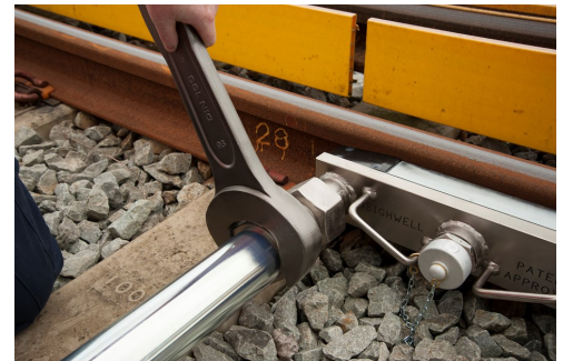
5. Securing the PTW into the track.
